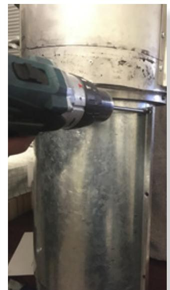
Flex collar and fit around the access panel. Socket the collar all the way up close to the air intake slots Ensure there is a rubber seal top and bottom of the collar.
