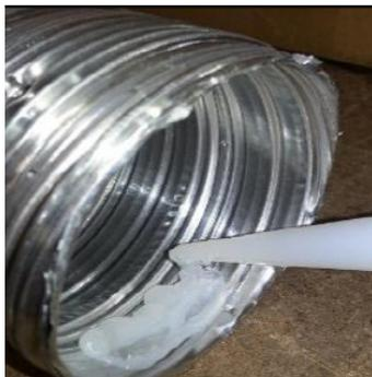
Apply sealant to flue inner and connector.
