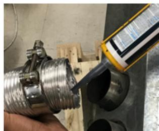
On the heater connection end - Fit clamp loosely & apply silicon inside the pipes. Apply an 8mm silicon bead fully around the inside of the flue and on the heater spigot. Smear the silicon around the spigot and pipe.
