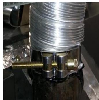
Slide flue onto connection spigot fully.
