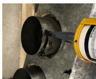
Recommended Silicon – Non-acetic, neutral cure 200°C or higher temperature rated. Bostik RTV 922 or similar.
