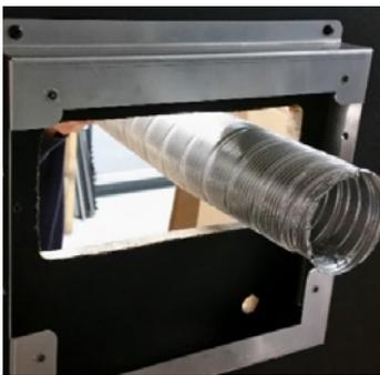
Cut air intake flue to length (Approximately 70mm through wall exit).
