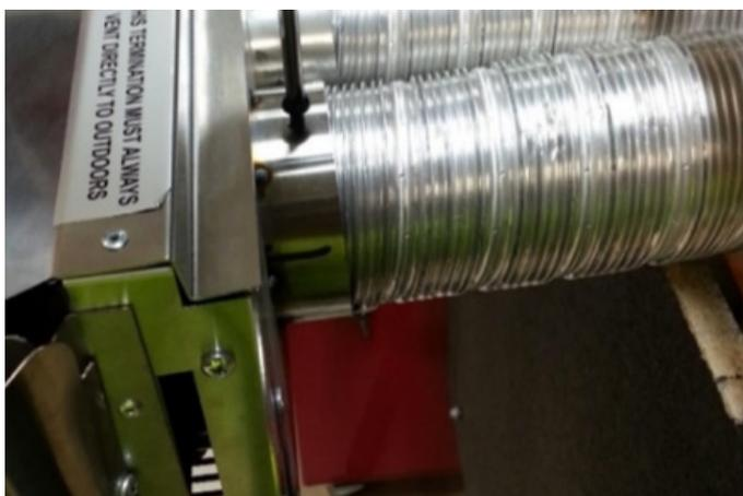
Cut inlet air tube. (Flue must extend a minimum of 50mm past the exit face of wall.) It is recommended that the intake tube is cut slightly longer and pushed back into wall upon fixing of wall terminal. Allow flue movement between terminal and last intake flue hanging clip.
