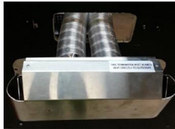
Push terminal into approximate position and affix onto wall.
