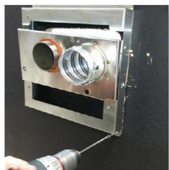
Locate wall mounting bracket into position and affix to wall.
