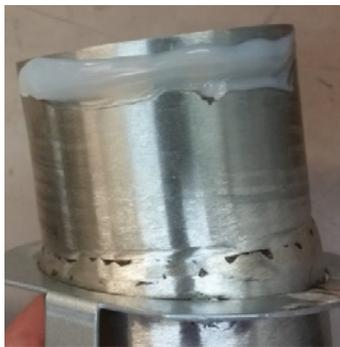
Apply sealant to flue inner and connector.
