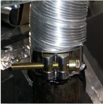
Slide flue onto connection spigot fully.
