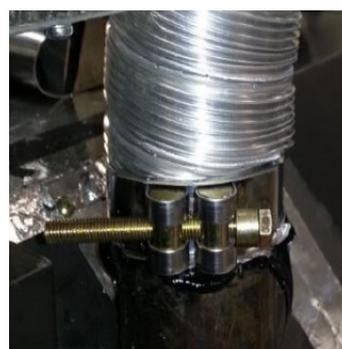
Slide flue onto connection spigot fully.
