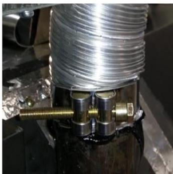
Slide flue onto connection spigot fully.
