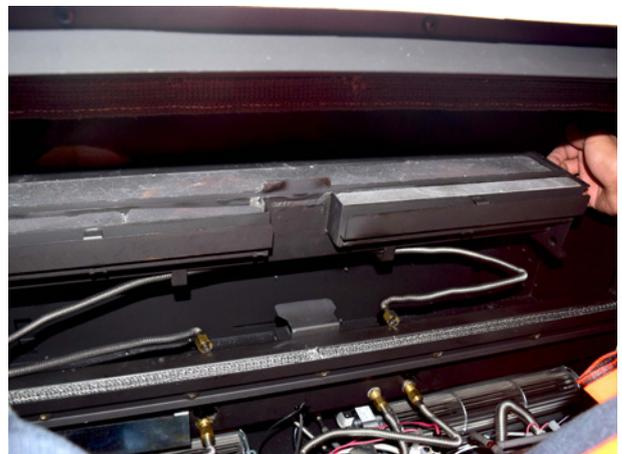
Undo wingnuts to remove burner and lift burner from position.
