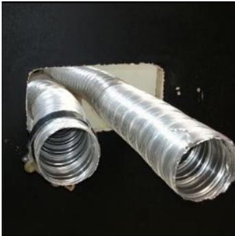
Cut flue exhaust tube (hot tube) to length (Approximately flush with wall exit). Connection plate will sit against wall.
