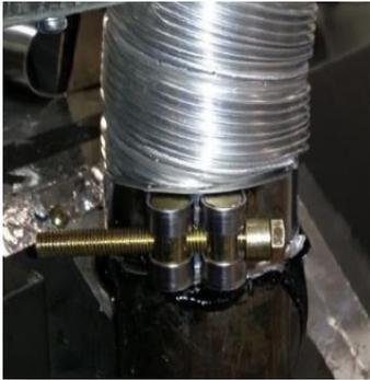
Slide flue onto connection spigot fully.
