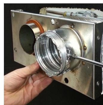
Feed air intake flue pipe through location spigot and fit retaining screw.
