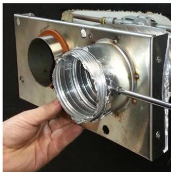
Ensure ends are burr free and round, test fit flue will slide over connection.
