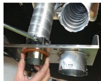
Slide flue onto connection spigot fully. Tighten clamp fully.
