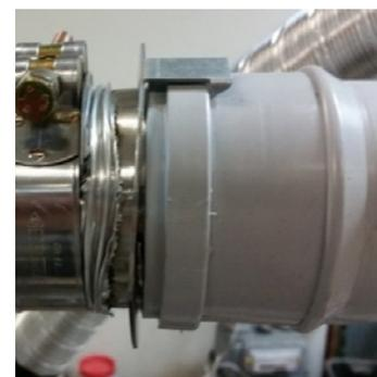
Apply soapy water to ring in Poly Pro flue and dampen surface of connector.
