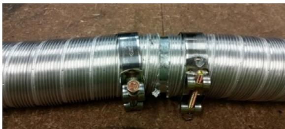
Slide each flue halfway onto connection joiner.
