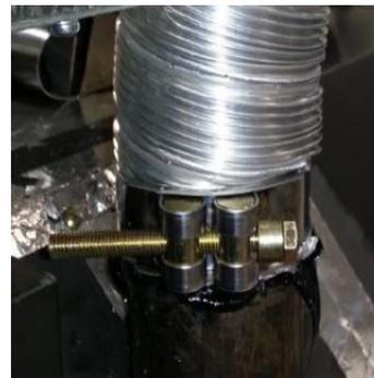
Slide flue onto connection spigot fully.
