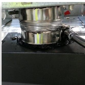
Fit flue exhaust insulation
