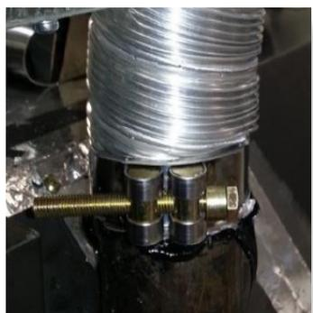
Slide flue onto connection pigot fully.
