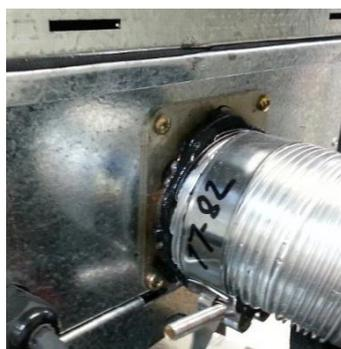
Slide flue onto connection spigot fully.
