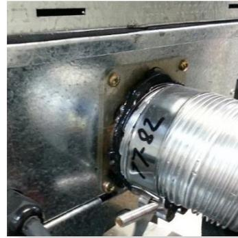
Slide flue onto connection spigot fully.
