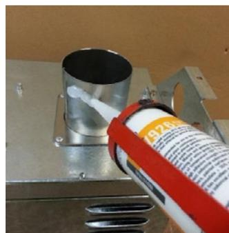
Apply an 8mm thick silicon bead fully around the lower fan connection spigot approx. 10mm from the end.
