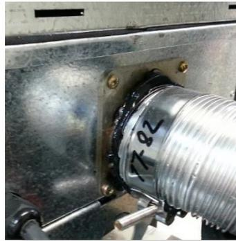
Slide flue onto connection spigot fully.
