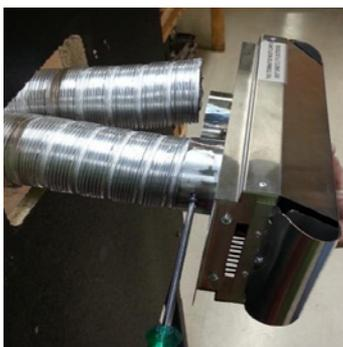
Feed hot exhaust flue into connection, ensure inserted 50mm. Fit retaining screw from below.
