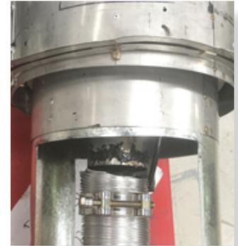
On the termination end - Fit clamp loosely & apply silicon inside the pipes. Apply an 8mm silicon bead fully around the inside of the flue and on the flue spigot. Smear smoothly around the surfaces.
