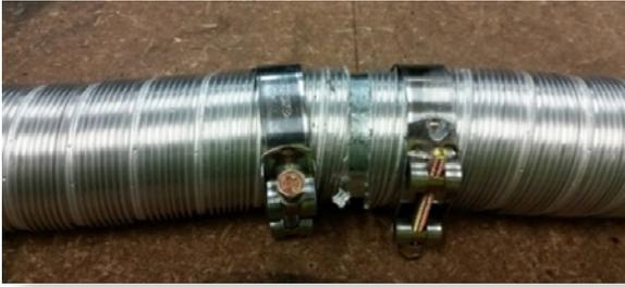
Slide each flue halfway onto connection joiner.
