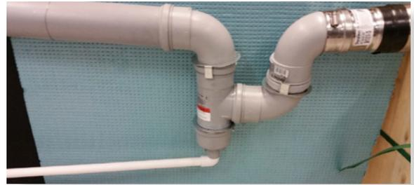
**NOTE** – DRAINAGE MUST FALL TOWARDS CONDENSATE TRAP LOCATED AT THE END OF THE ALUMINUM FLUE SECTION
