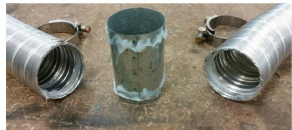
Apply an 8mm thick silicon bead fully around both ends of connector approx. 10mm from the ends.
