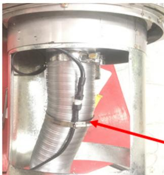
Connect the fan power cable from the appliance to the termination.
