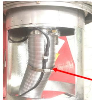
Connect the fan power cable from the appliance to the termination.
