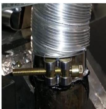
Slide flue onto connection spigot fully.
