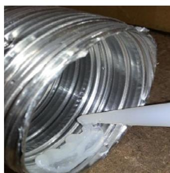
Apply an 8mm silicon bead fully around the inside of the flue end, both ends.
