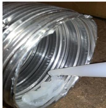
Flexi flue is in 7m lengths. A maximum of 2 lengths can be used.
