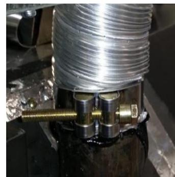
Slide flue onto connection spigot fully.
