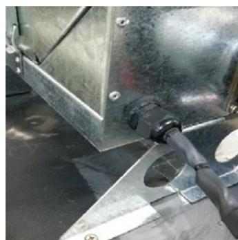
Fit 2nd flue clamp loosely onto the 65mm section of flue.
