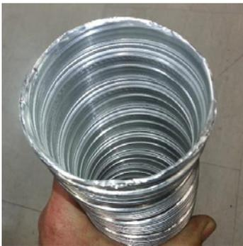
Cut flue to length to suit connection. Ensure ends are burr free and round, test fit flue will fit over connection.
