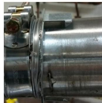
Fit flue clamp over flue (loosely).
