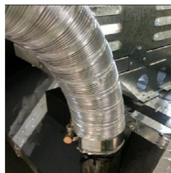
Clip flues as required to provide adequate support.
