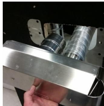
Assemble condensate drain and attach to pipe exiting wall. PVC pressure pipe cement must be used.
