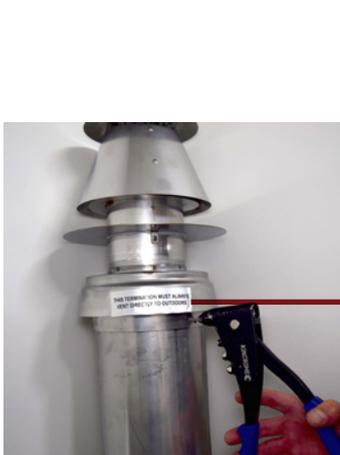
Screw or rivet in 3 places to hold in place.
