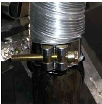
Repeat for air intake flue connection.
