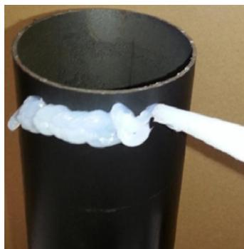
Apply an 8mm thick silicon bead fully around heater connection approx. 10mm from the top.
