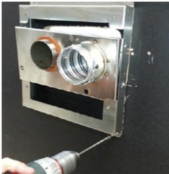
Locate wall mounting bracket into position and affix to wall.
