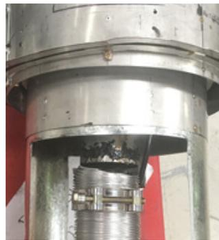
On the termination end - Fit clamp loosely & apply silicon inside the pipes. Apply an 8mm silicon bead fully around the inside of the flue and on the flue spigot. Smear smoothly around the surfaces.
