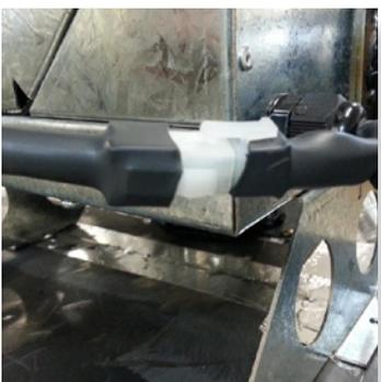
Connect power lead to fan module. Ensure lead is clipped to support where required.
