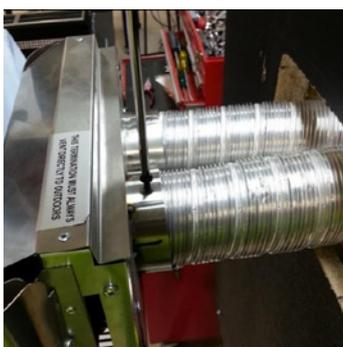
Feed air intake flue into connection, ensure inserted 50mm. Fit retaining screw from below.
