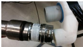
Apply soapy water to the fitting and to the connection on the rooftop termination
