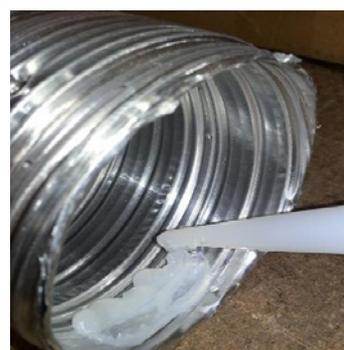
Apply an 8mm silicon bead fully around the inside of the flue end
