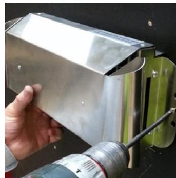
**Setup with internal fan module with wall termination – mid flue mounted**
