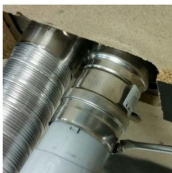
Push terminal into approximate position and affix onto wall
