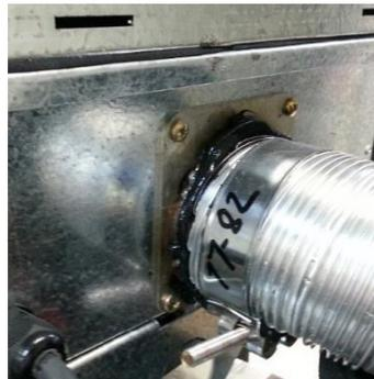
Slide flue onto connection spigot fully.
