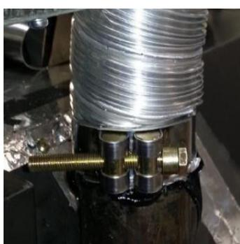
Slide flue onto connection spigot fully.
