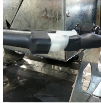
6. Connect power lead to fan module. Ensure lead is clipped to support where required.
