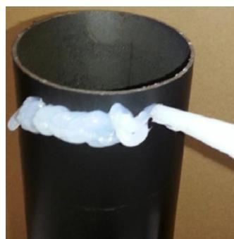
Recommended Silicon – Non-acetic, neutral cure 150degc or higher temperature rated. Bostik RTV 926 or similar.
