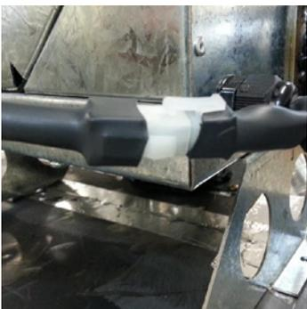
5. Connect power lead to fan module. Ensure lead is clipped to support where required.
