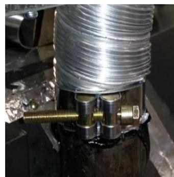
Slide flue onto connection spigot fully.
