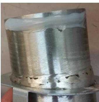
Apply sealant to flue inner and connector.
