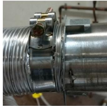
Fit flue clamp over flue (loosely).
