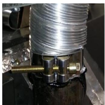
Slide flue onto connection pigot fully.
