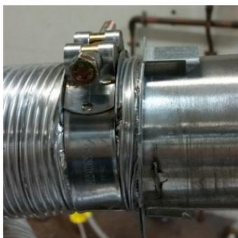
Fit flue clamp over flue (loosely).
