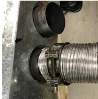
Slide flue onto connection spigot fully. Tighten clamp fully. Wipe excess silicon, visually check connection to ensure connection is fully sealed.
