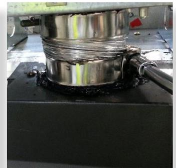
Where fan sits higher, ensure fan assembly is supported on a frame. Where timber framing is used clearances to flue and fan box must be maintained.
