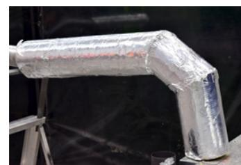
Bends were practical should be insulated, by cutting the insulation into segments and taping together.
