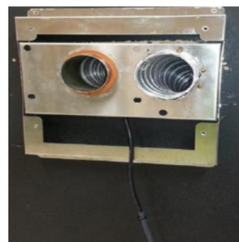
Feed power cable through bottom area of bracket.
