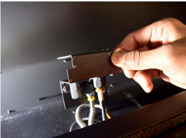
Remove pilot orifice from pilot or replace whole pilot assembly with correct gas type.
