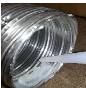
Apply an 8mm thick silicon bead fully around heater connection approx. 10mm from the top.
