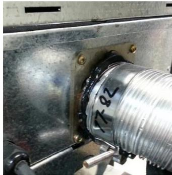
Slide flue onto connection spigot fully.
