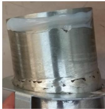
Apply sealant to flue inner and connector.
