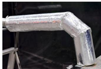
Bends were practical should be insulated, by cutting the insulation into segments and taping together.
