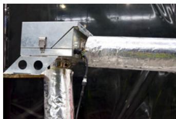
Insulation must be fitted prior and after the inline powerflue fan.
