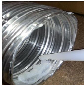
Apply an 8mm silicon bead fully around the inside of the flue end (heater connection end)
