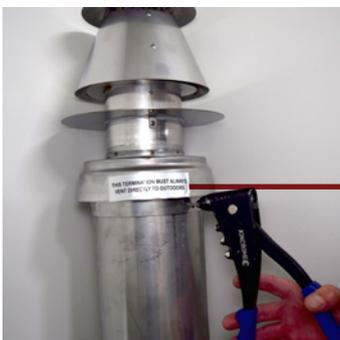
**IMPORTANT-** Apply silicon bead between inner connection of cowl and flue pipe to seal inner flue to cowl. Outer does not require sealing.
