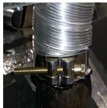
Slide flue onto connection spigot fully.
