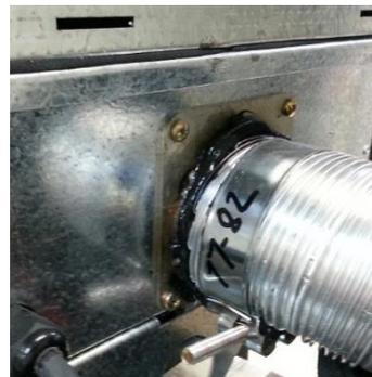
Slide flue onto connection spigot fully.
