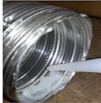
Apply sealant to flue inner and connector.
