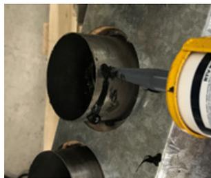
On the heater connection end - Fit clamp loosely & apply silicon inside the pipes. Apply an 8mm silicon bead fully around the inside of the flue and on the heater spigot. Smear the silicon around the spigot and pipe.
