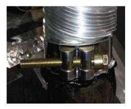
Slide flue onto connection spigot fully.
