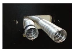
Cut flue exhaust tube (hot tube) to length (approximately flush with wall exit). Wall termination will sit against wall.
