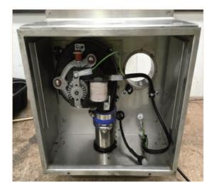
Feed power cable through wall and into wall terminal.
